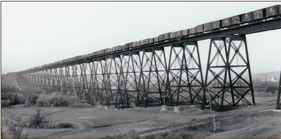
Railroad trestle crossing Sheyenne at Valley City
